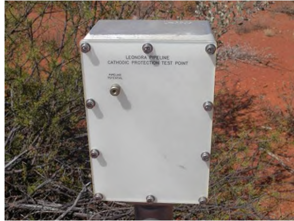
Photograph 4 Cathodic Protection along Pipeline Route
