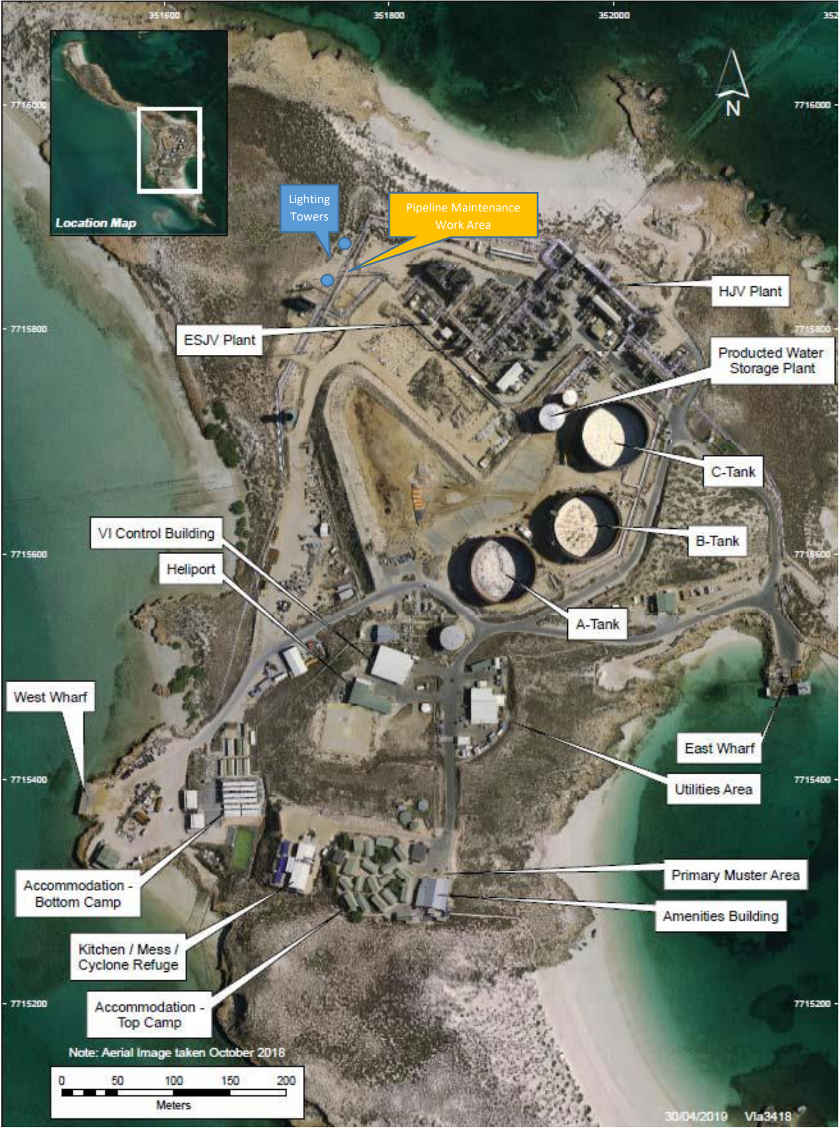
Figure 4-1: Pipeline maintenance work area and proposed location of lighting towers
